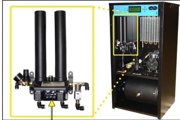
**9.9.3** Use a Voltmeter to measure the DC voltage across each set of “VALVE” terminals.
